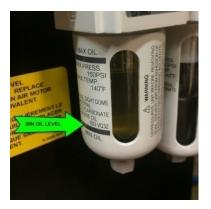
**NOTE:** Failure to maintain oil level in lubricator will **void warranty** of all pneumatic components.
